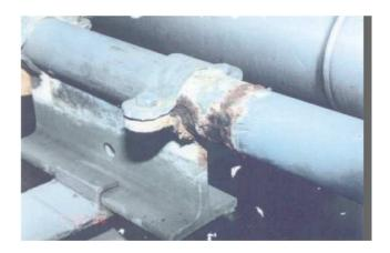
Plant and equipment must be designed to allow for effective sealing of the insulation system
